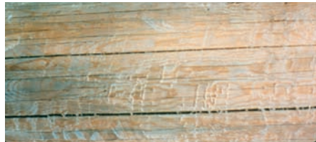
Felted wood after power washing.
