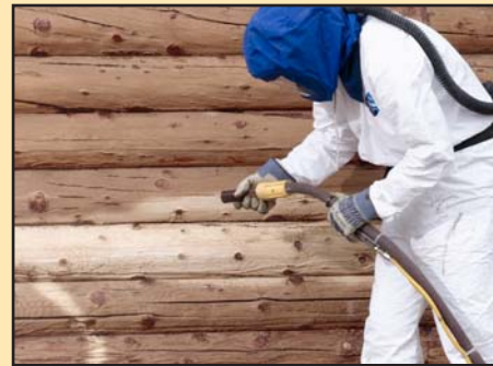
Corn Cob Blasting (Recommended method)
