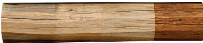
Prep method used was power washing followed by an Osborn Brush. The bare wood shown in the middle DOESN'T return to its natural color after pressure washing.
