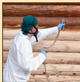
Spray on stain.
